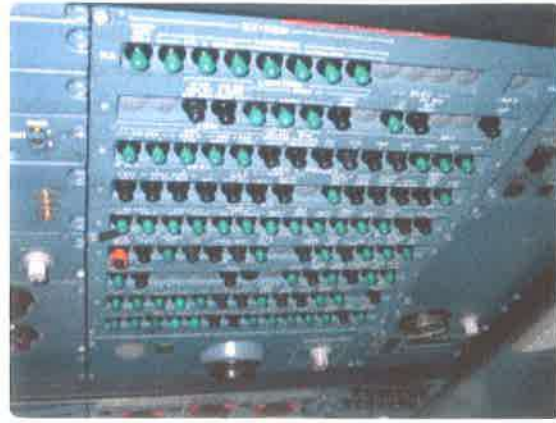
Figure 8-31. Circuit breaker panel.
