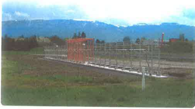
Figure 7-106. An ILS localizer antenna.
