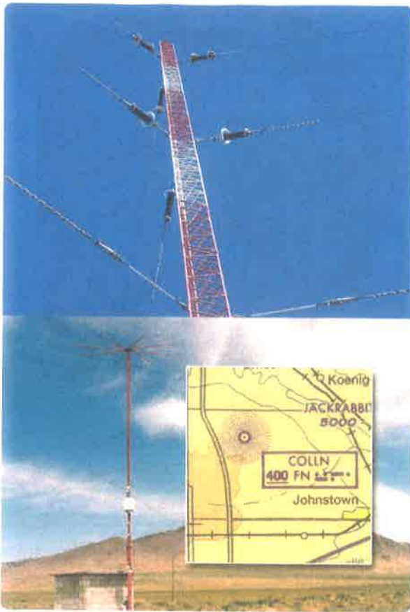
Figure 7-102. Non-directional broadcast antenna.
